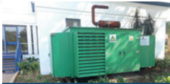
The standby generator
